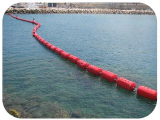
The barriers consist of individual modules joined together with galvanized chain and clamps.
