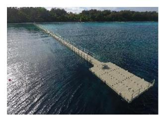
RotoDock HDPE pontoon modules create a robust, stable and versatile pontoon system that is virtually maintenance free.
